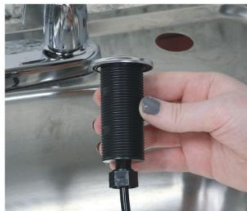
Remove Nut & Washer & Connect Hose
